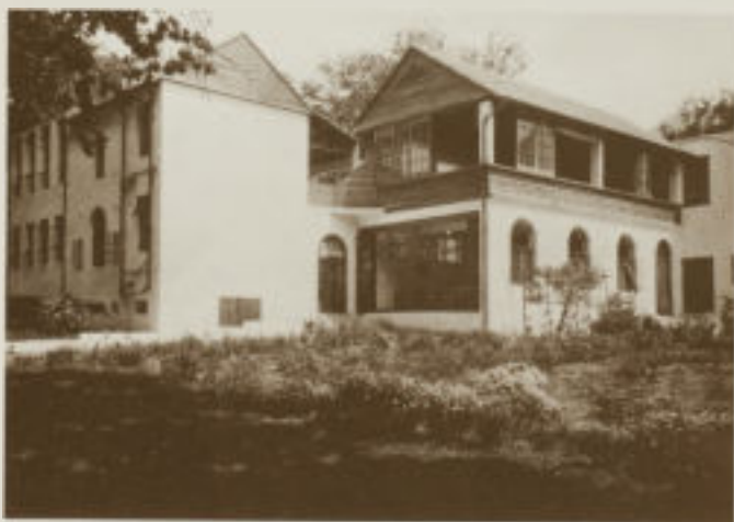
The 1929/1930 Extensions: the new Dining Room on the right has an open sleeping balcony above it, while the wing on the left comprises new classrooms. The narrow open sleeping balconies had some sliding windows, but with the passage of years, they mostly became immovable as they warped and stuck fast.
