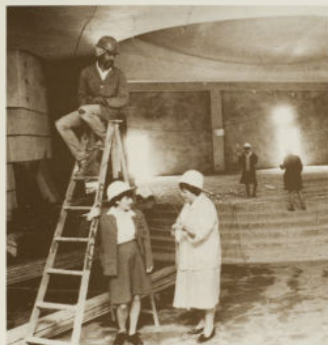
The new Theatre being built in 1988. Mrs Chris Brathwaite (in charge of fundraising) and Headgirl Keshya Maseti check the progress.
